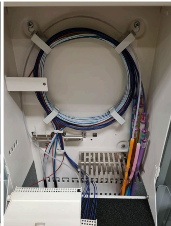
Route the tube the desired way towards the splice cassette
