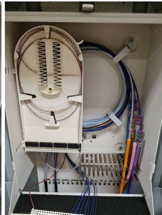
Route the tube the desired way towards the splice cassette
