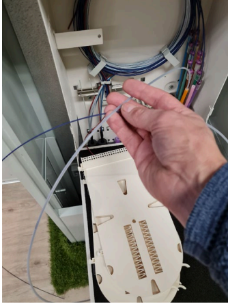
Push a predefined length of 3mm tube onto the Stingray unit
