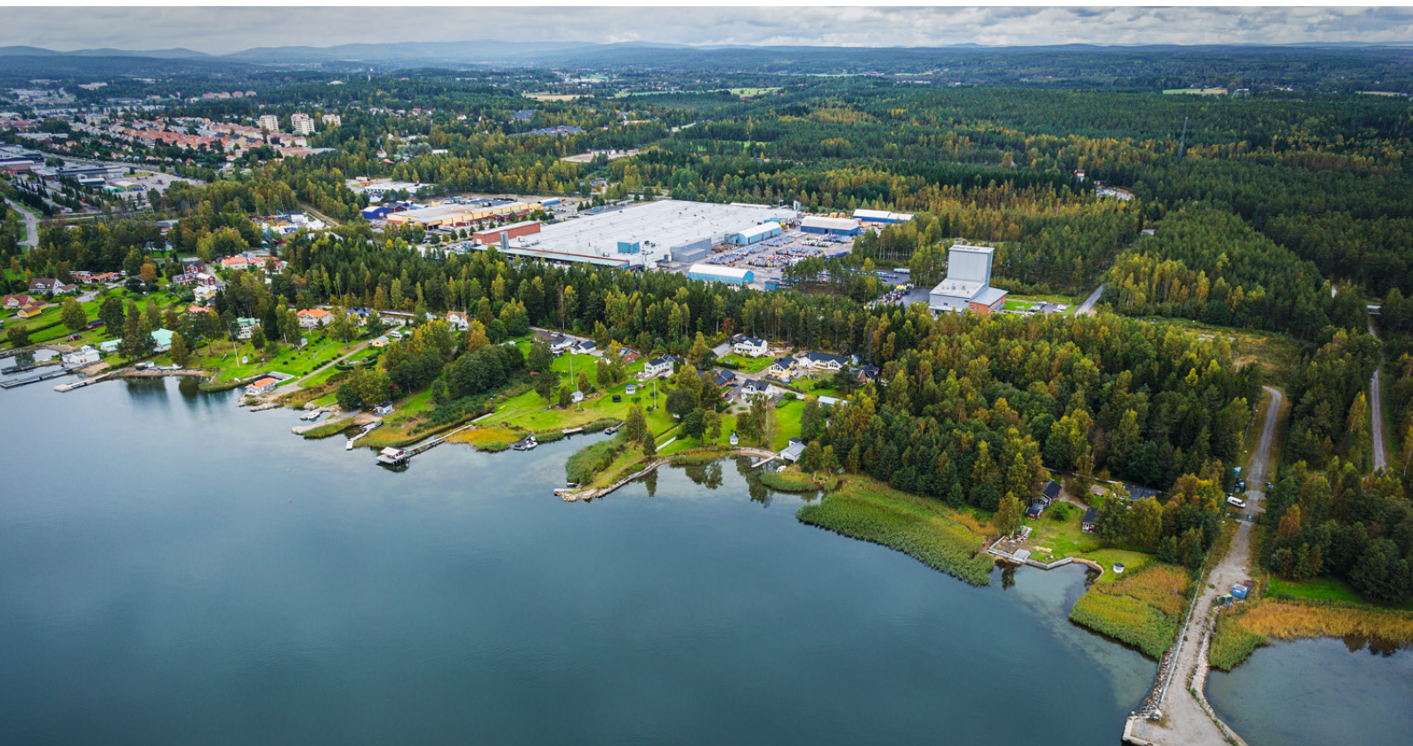
Hexatronic Cables & Interconnect AB i Hudiksvall
