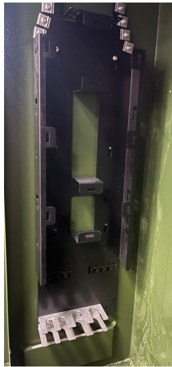
Position the Mid-span unit and install top two screws loosely
