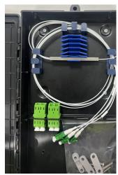
6. Remove the dust caps from the adapter and the splitter tail, then carefully install by plugging in till you hear the click. Repeat for each splitter tail.
