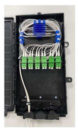
14. Splice pigtails to the fibres in the next box and then the splitter as normal.
