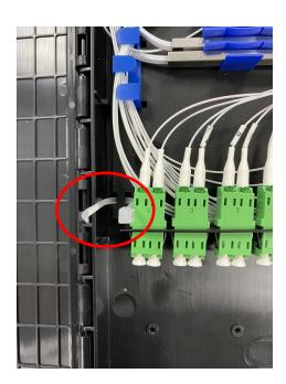
11. Mid span required is 1.4m dress the cable and mark your input side as shown.
