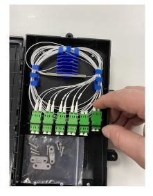
4. Install the splitter into the holder as shown making sure to orientate it correctly. The 8 tails will exit the holder to the left and the single feed to the right.
