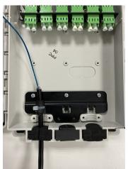
2. Install cable tie to tray area in (red circle) and fit foam tape at the anchor point to the buffer tube.
