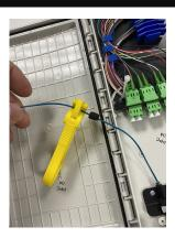
4. Install the buffer tube into the cable tie clamping on the foam tape .(Note do not Over tighten this is only to hold the tube loosely so it does not move).
